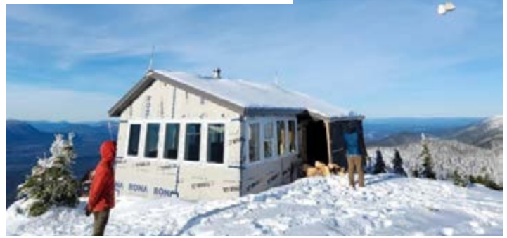
under construction in 2024
