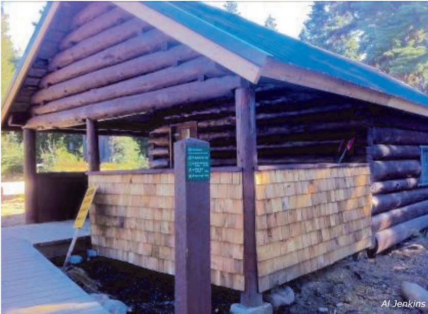
Refurbished Taylor Cabin
