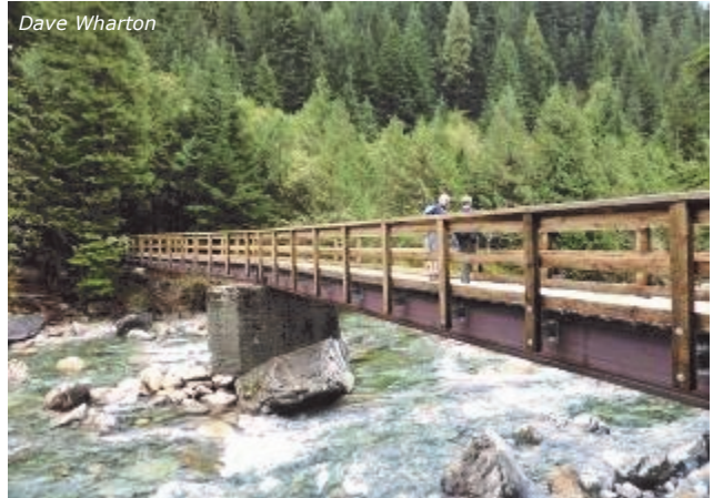
New bridge over Gold Creek links East and West Canyon Trails
