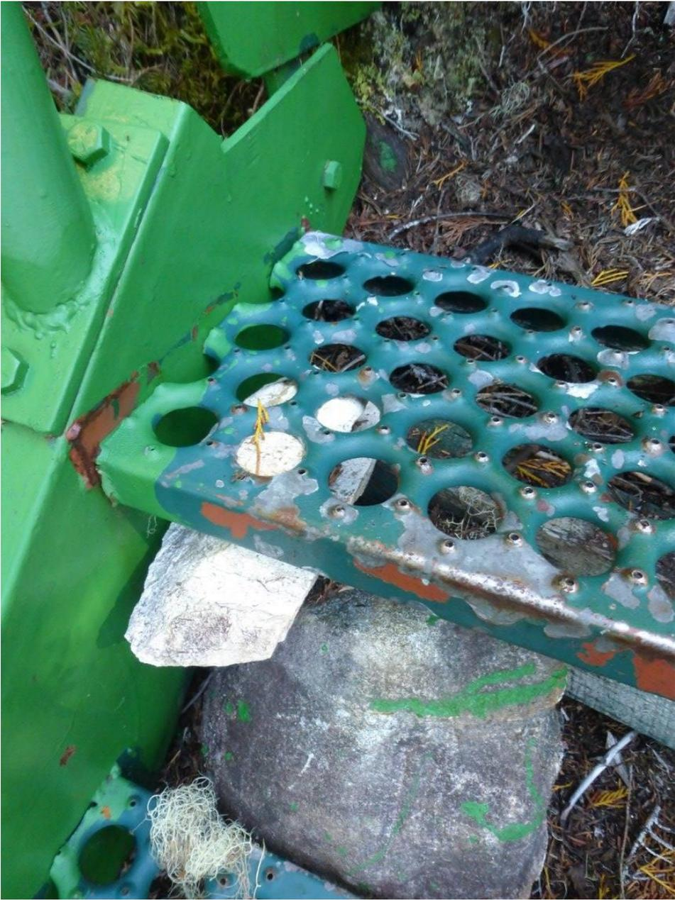
The metal staircase on the Bedwell Trail has a broken step from the welds breaking. It has been temporarily band-aided with a piece of wood used to brace the step and g-clamps holding it into place. It is structurally unsafe.
